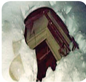
The picture on the left shows properly gridded skylights to prevent workers from falling through multiple skylights. The picture on the right shows an unprotected skylight that resulted in a tragic and fatal incident.
