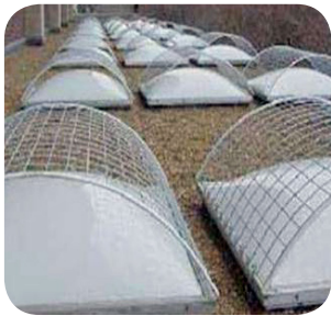
The picture on the left shows properly gridded skylights to prevent workers from falling through multiple skylights. The picture on the right shows an unprotected skylight that resulted in a tragic and fatal incident.
